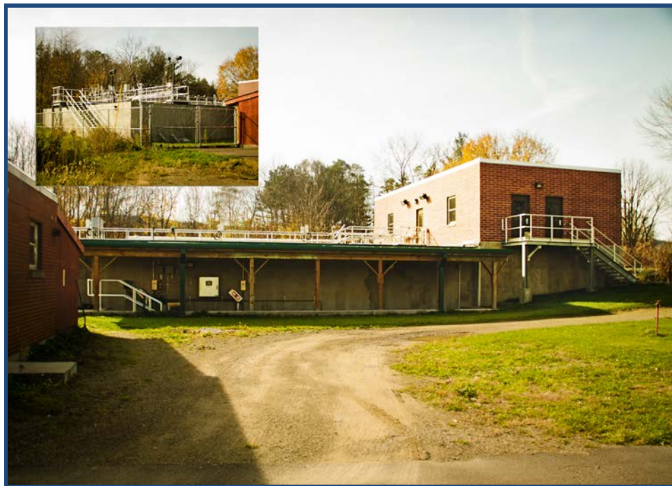
Belmont Water Treatment Plant
