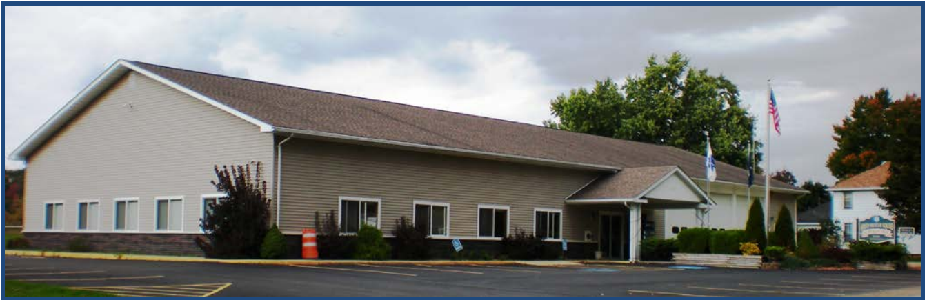
Amity Rescue Squad Facility
