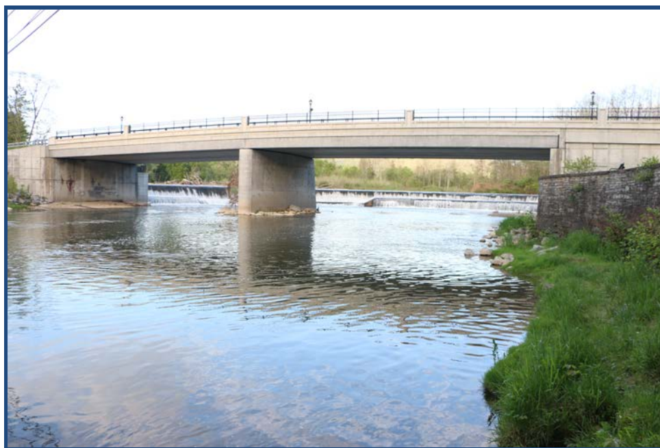
NY State Route 19 Bridge over the Genesee River Falls and Dam
