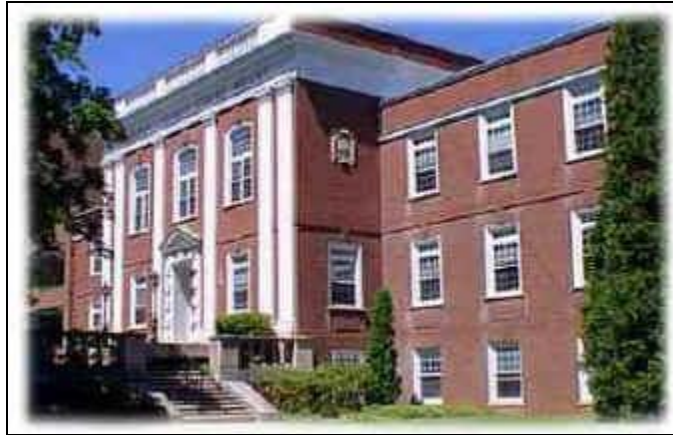
Allegheny County Courthouse in Belmont
